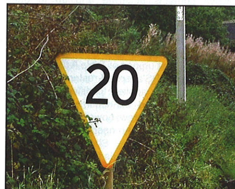
The Mark II version of the Morpeth Board, introduced after the second Morpeth derailment, has improved visibility.
