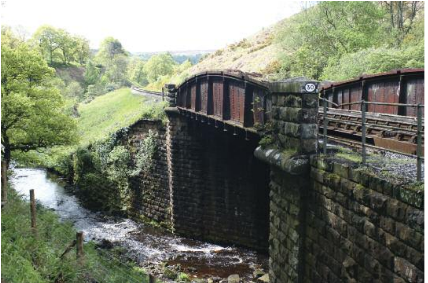
View looking towards Grosmont in June 2009. Note the substantial masonry wing walls supporting the railway on either side of the bridge in addition to the substantial abutments.
