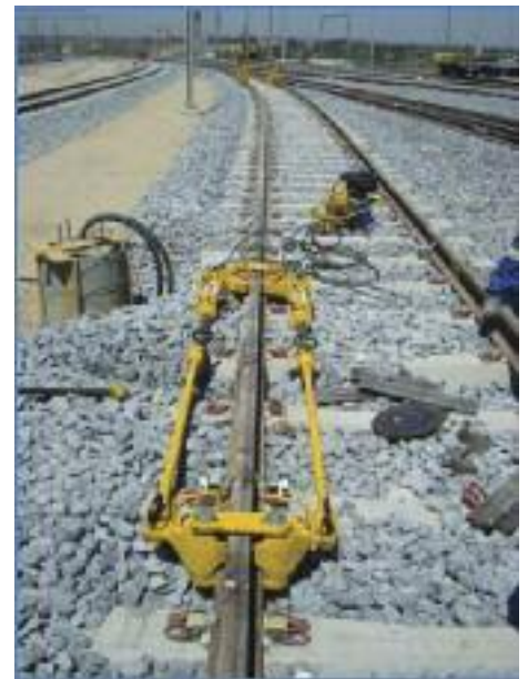
Figure 7: Tensioner kept in place after destressing waiting for the thermit weld to cool down
