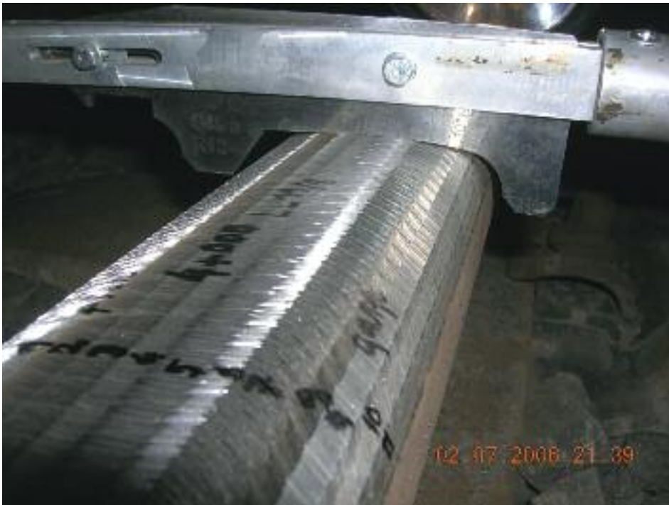
Figure 8: Figure 7 curve end; after grinding with 7 passes; desired profile done. Figure 7-8 photos are belonging to Izmir Metro archive.
