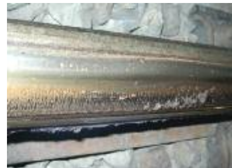
Figure 4 ; Before and after rail grinding results
