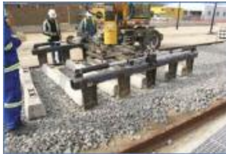
Figure 3: Sleepers being placed
