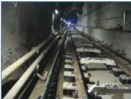
Figure 9: Slab track ready to be covered prior to concrete pouring
