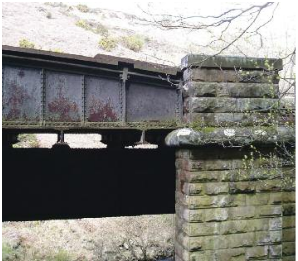
The Goathland end of the Down side outer main girder showing the underslung cross girders and the centre girder added in 1908. Note also the steel strengthening fitted to the cast iron top flange in 1906.
