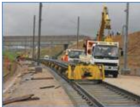
Figure 4: Rail train on its way to be off-loaded
