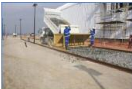
Figure 2: Placing bottom ballast
