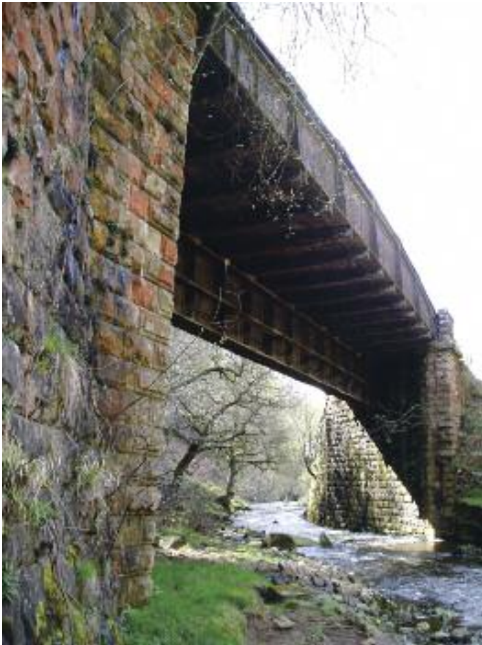
The North or Up side of the bridge showing the centre girder and the skew. The space between the abutments and under the bridge appears excessive for the size of the Eller Beck River flowing through!
