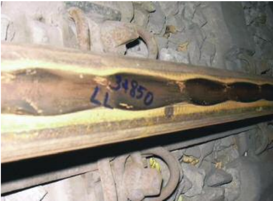
Figure7. 100 mm short waves where on clotoid to curve, r=400 m, cant=50 mm before grinding monitoring
