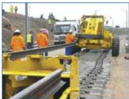
Figure 5: Rail string pulled from rail train onto the sleepers
