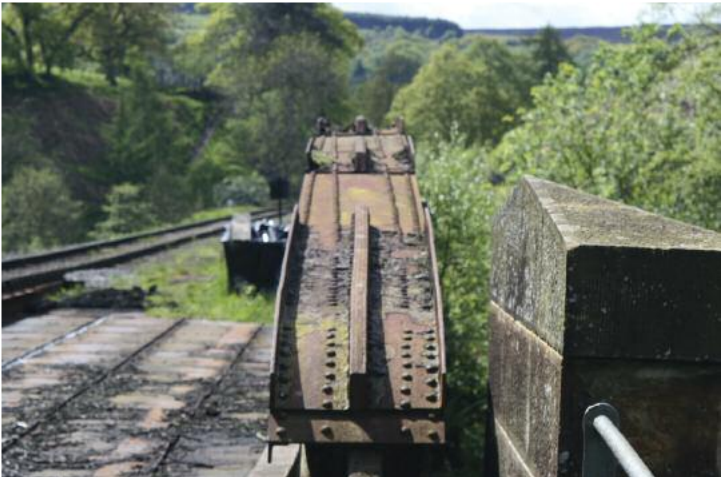
The Goathland end of the Up side main girder showing the steel strengthening added in 1906. Note the uneven lines of rivets are not parallel due to the distortion in the original main girder.
