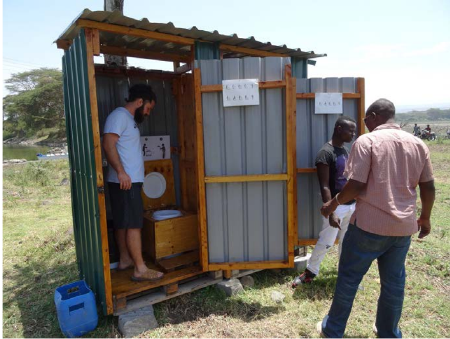
Figure 7-Compost toilets at Lake Naivasha, Kenya.
