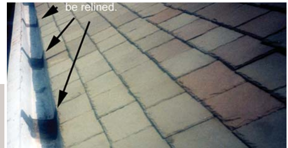
Figure 25 (above): Box gutters require expansion joints, otherwise the solder joints will crack under pressure. This is evident by solder joints that have been covered by roof cement, a common sight on box gutters, new and old.
