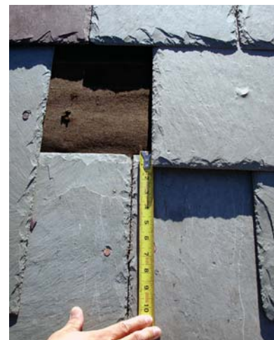
Figure 9 (above): Headlap is a critical detail on a slate roof. Lack of headlap will cause an entire roof to be condemned. Read more about headlap in TR6.
