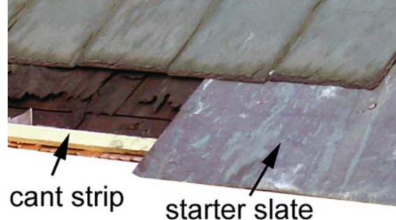
Figure 7 (above): Note that the starter slate is laid back-side-up and is propped up by a cant strip.
