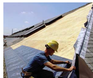
Figure 4: Traditional slate roofing systems, despite their incredibly successful performance, are being largely abandoned in favor of plywood roofs with peel and stick underlayment.
