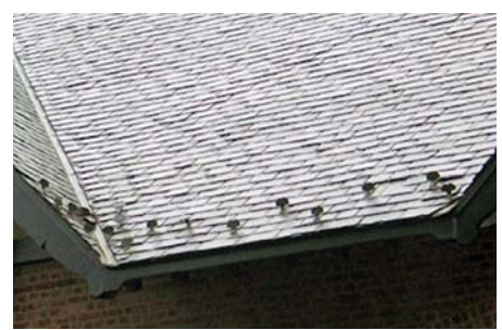
Figure 32: Snowguards must be installed in adequate quantities, or else they will get knocked off in the first bad ice storm and will damage the roof in the process.
