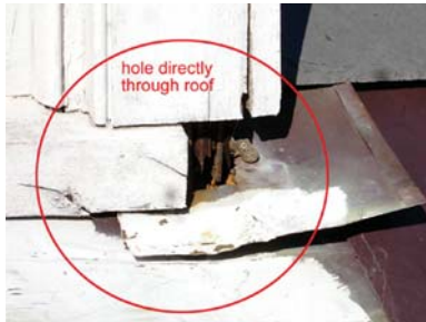
Figure 24 (above): This is a case where the corner flashing is neither folded nor soldered, leaving a large hole in the roof.
