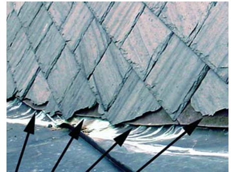
Figure 34: Slate roofing requires the correct tools to do the job right. There is no excuse for the sort of work shown above.
