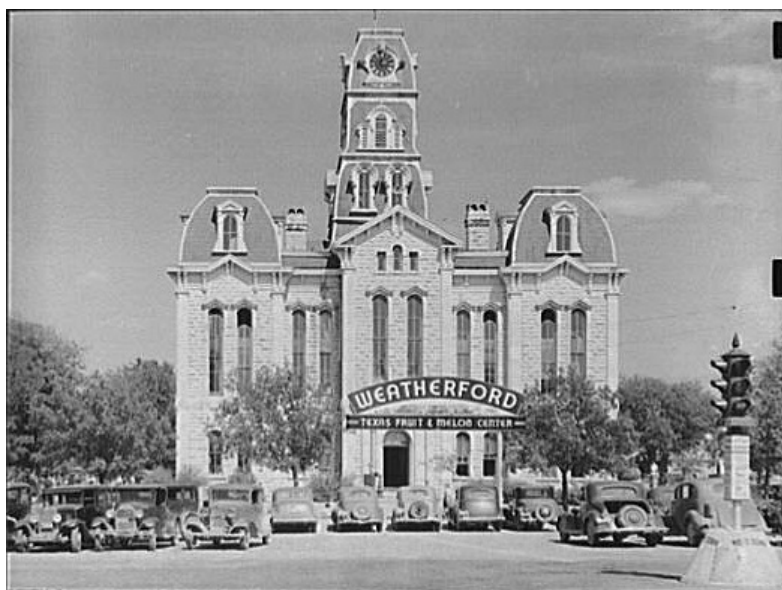
Period sedans in front of the Weatherford courthouse in 1939. Weatherford is less than ten miles southeast of Howard's birthplace of Peaster. Library of Congress, Prints & Photographs Division, FSA-OWI Collection
