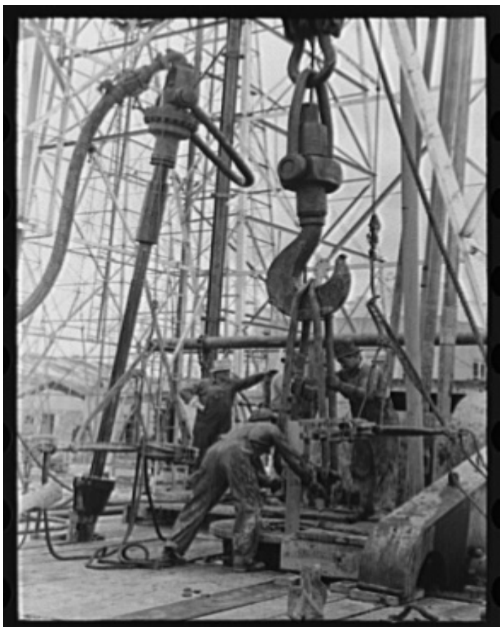
Activity at oil well showing one length of pipe resting on the kelly joint into the rat hole with operations for removing other lengths of pipe from the hole. Oil well, Kilgore, Texas. 1939.
