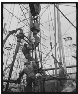
Activity at oil well showing one length of pipe resting on the kelly joint into the rat hole with operations for removing other lengths of pipe from the hole. Oil well, Kilgore, Texas. 1939.
