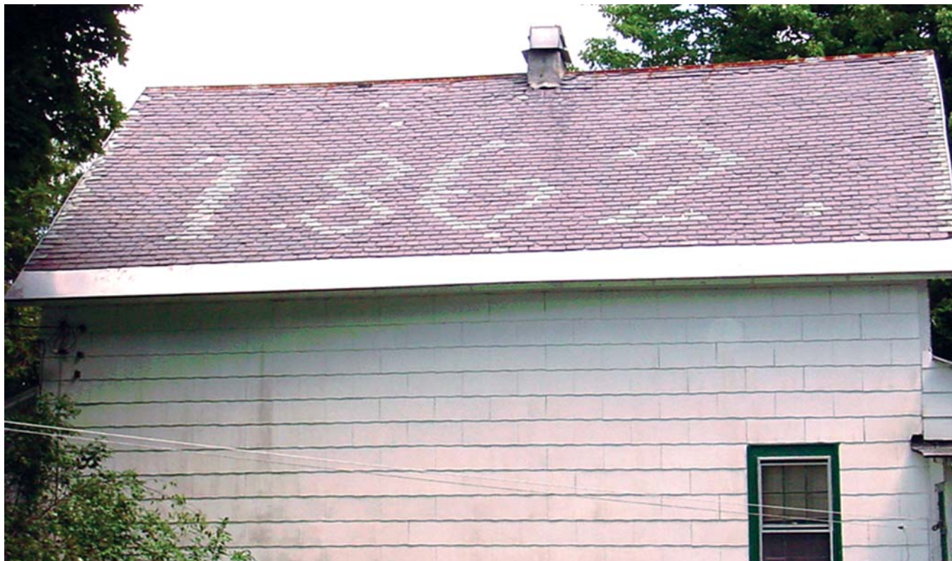
▲ The 1862 roof located in western Vermont has a VT unfading green slate inscription on a VT purple slate roof — thinly split stone nailed to a one inch thick board roof deck — a roofing system easily replicable today.
