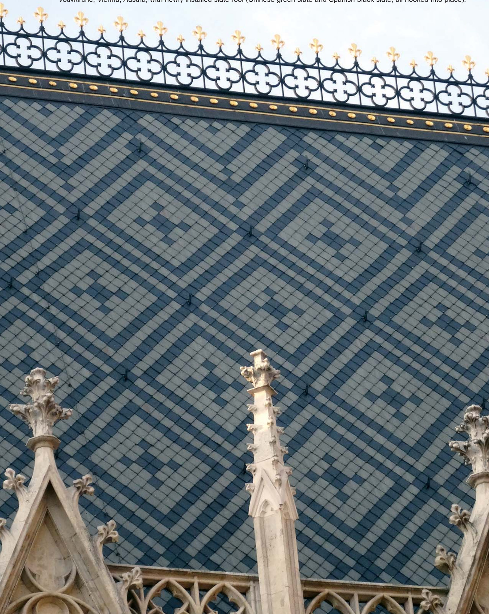
Votivkirche, Vienna, Austria, with newly installed slate roof (Chinese green slate and Spanish black slate, all hooked into place).
