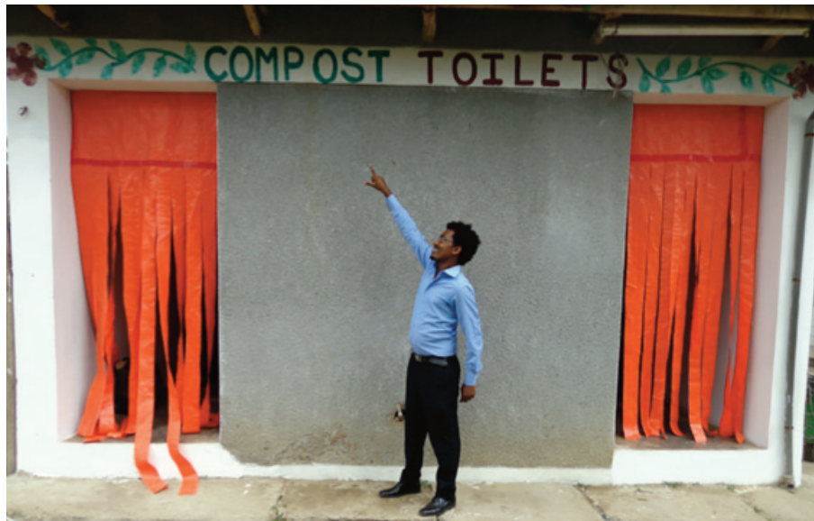
This is a compost toilet building at the Ayder Referral Hospital & medical school, Mekelle, Tigray, Ethiopia.
